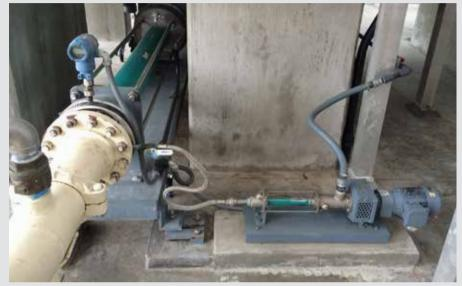
Polymer injection - NETZSCH FLR system reduces friction losses
